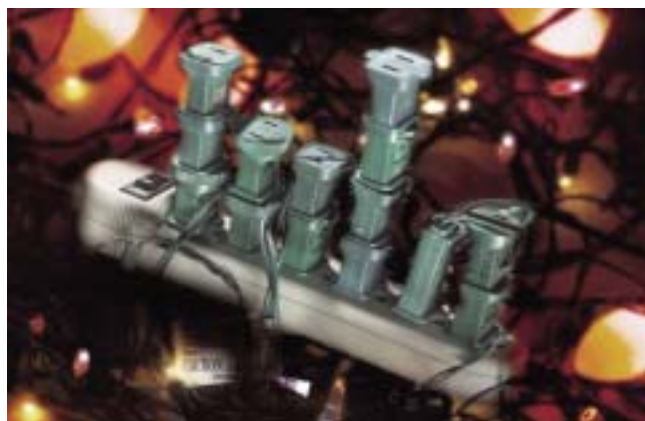
Don't overload extension cords with too many sets of lights.
